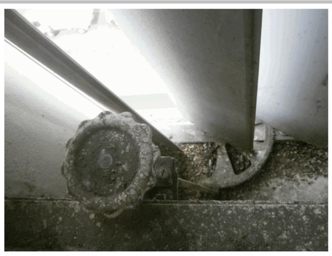
Internal detail of original aluminium louvre mechanism Caption:
